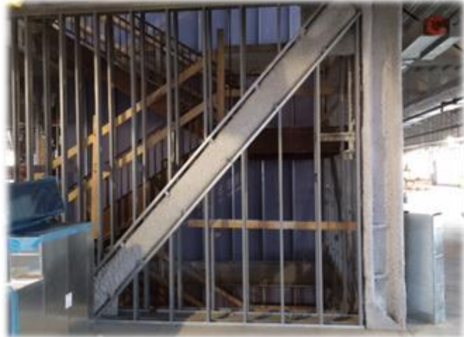
Figure 26 Stud Framing for Drywall Placement (Image Courtesy of David Walenga)
