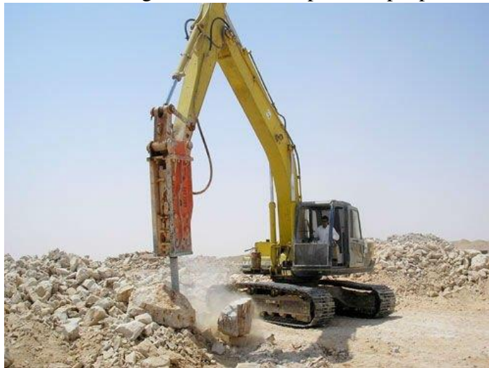
Figure 55 Traditional Rock Excavation Utilizing a Hammer Attachment
