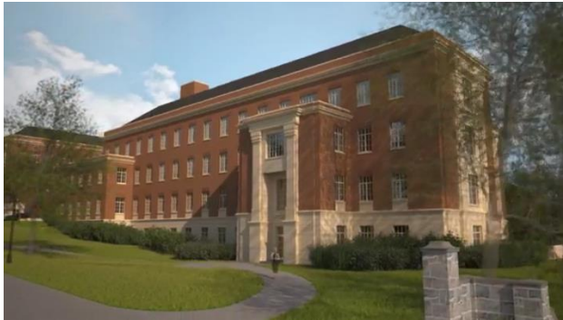
Figure 11 HHD Building Facing West. Exterior Masonry Designed to Match That of Surrounding Buildings
